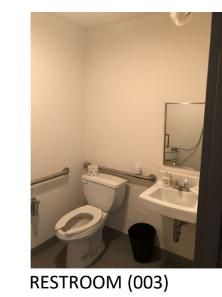
1 RESTROOM COMPLIANCE (PHOTOS) NOT TO SCALE
