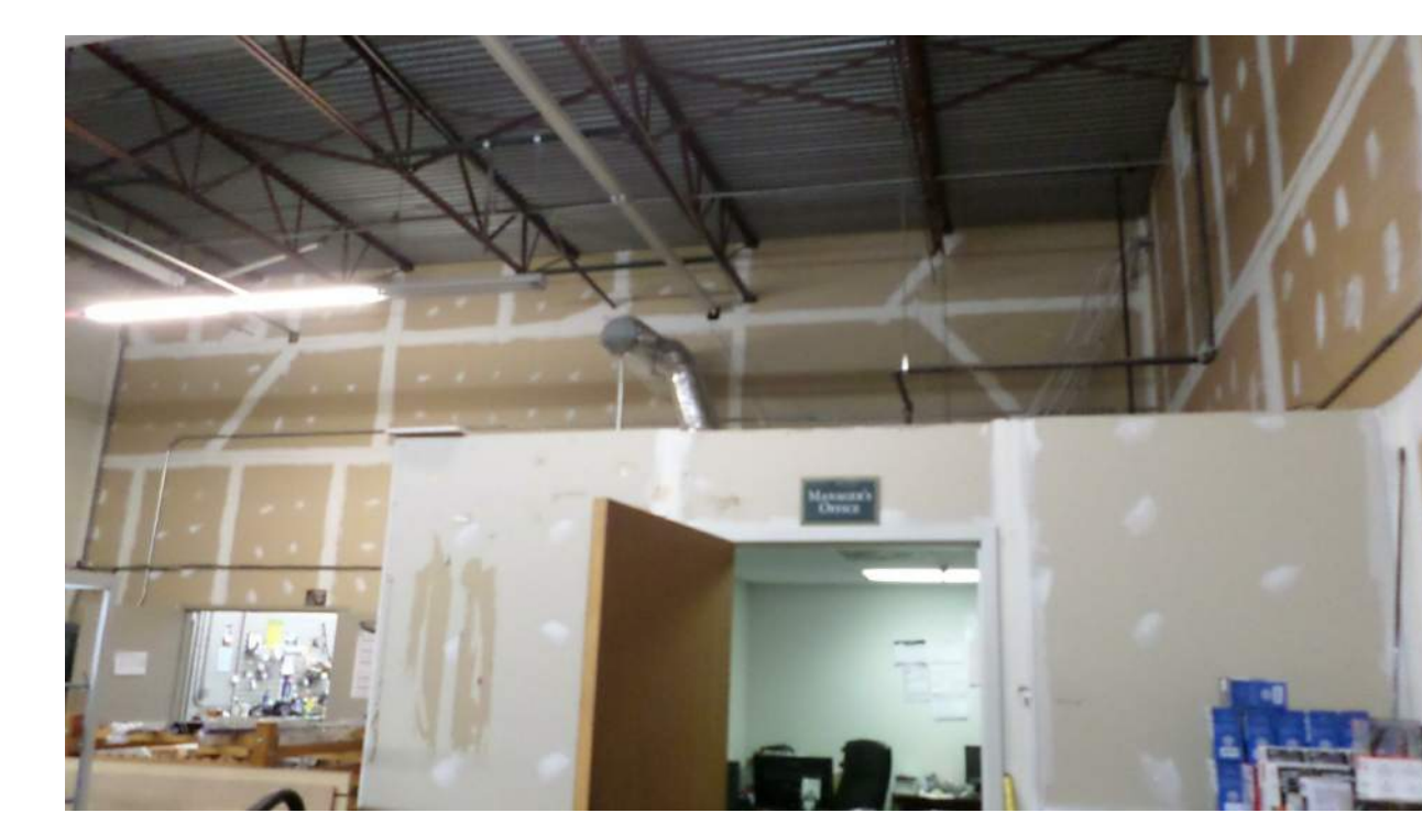
VIEW OF REAR INTERIOR - FACING SOUTH WEST.
