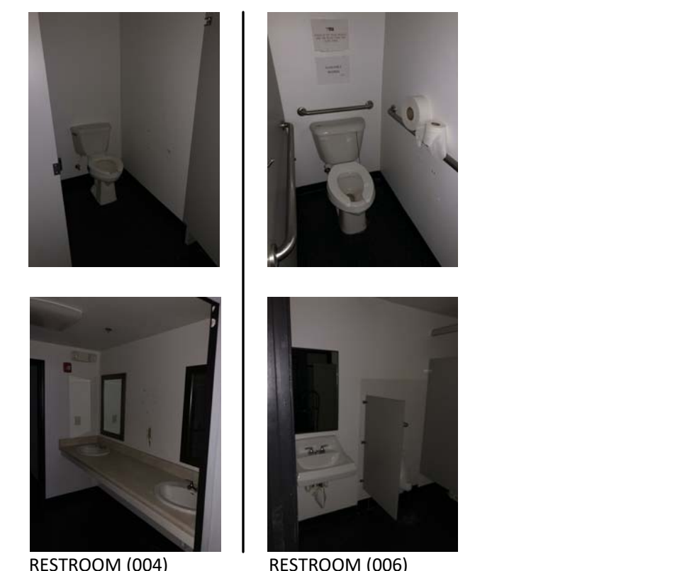
1 RESTROOM COMPLIANCE (PHOTOS) NOT TO SCALE
