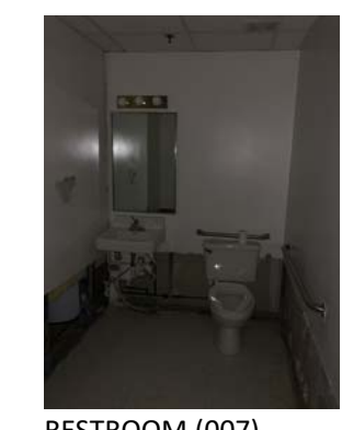
1 RESTROOM COMPLIANCE (PHOTOS) NOT TO SCALE
